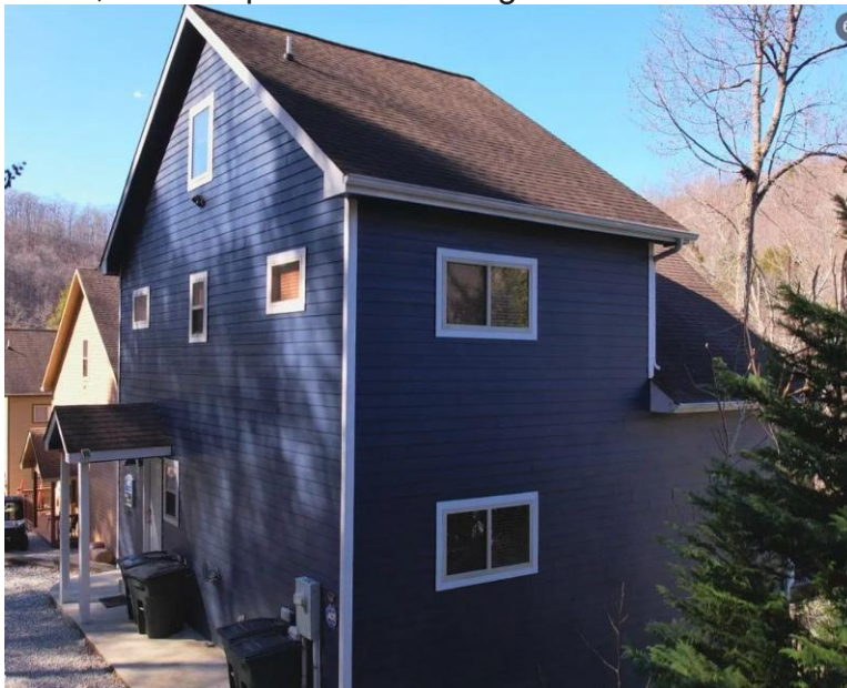
Figure 3. Front door and exterior of single-family RESIDENTIAL home at [REDACTED]
