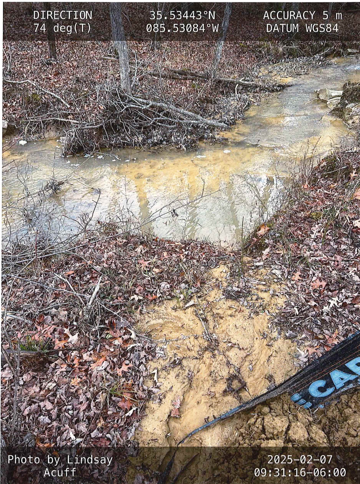
Photo 5: Further sediment entering waters of the state, silt fence overtopped.
