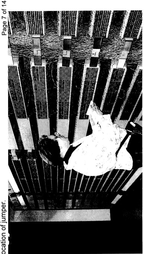
Step 8: Technician locates and removes end of jumper connected to the BellSouth cable pair.
