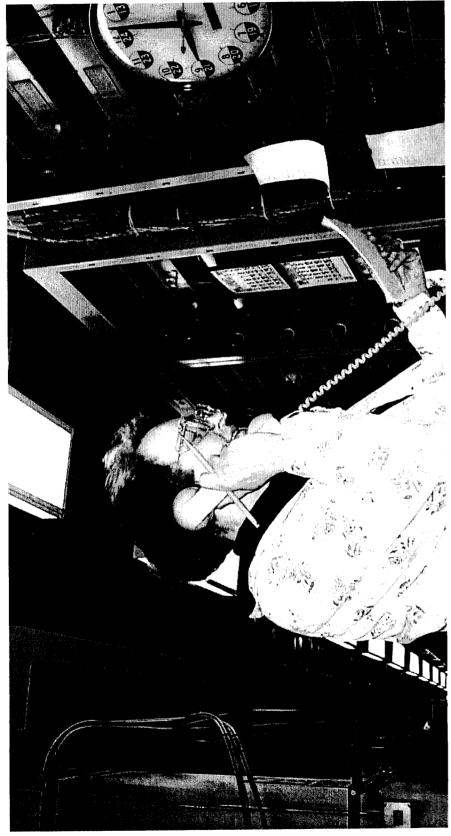
Step 5: Technician conducts ANAC test to verify that correct loop is being cutover.
