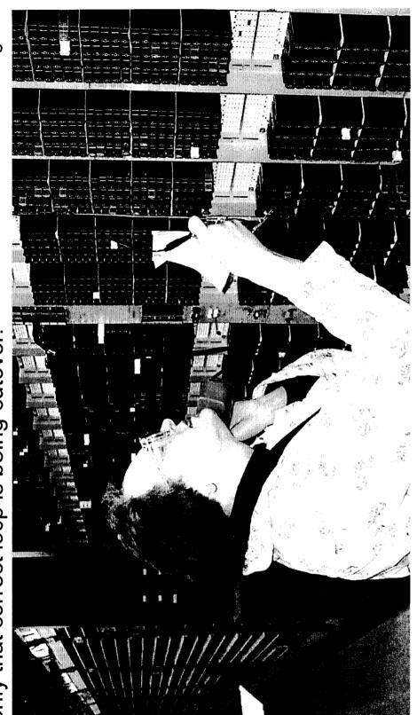
Step 6: Technician walks along Main Distributing Frame to locate both ends of jumper to be cut.
