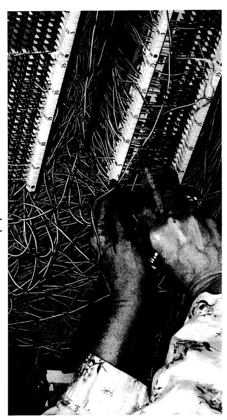
Step 13: Technician conducts ANAC test to verify that loop has been cut to correct CLEC switch port.
