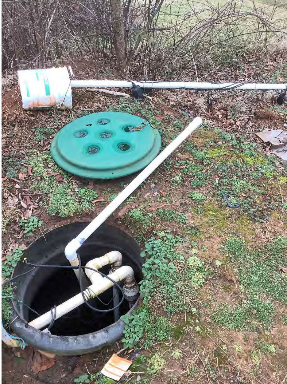
X2. Wastewater effluent being directed to adjacent ditch rather than the drip field.
