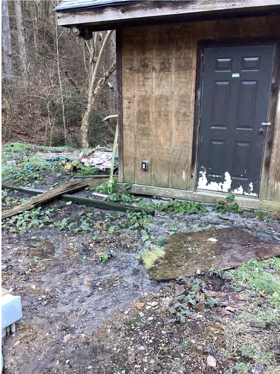
X2. Wastewater effluent being discharged from the control building rather than to the drip field.
