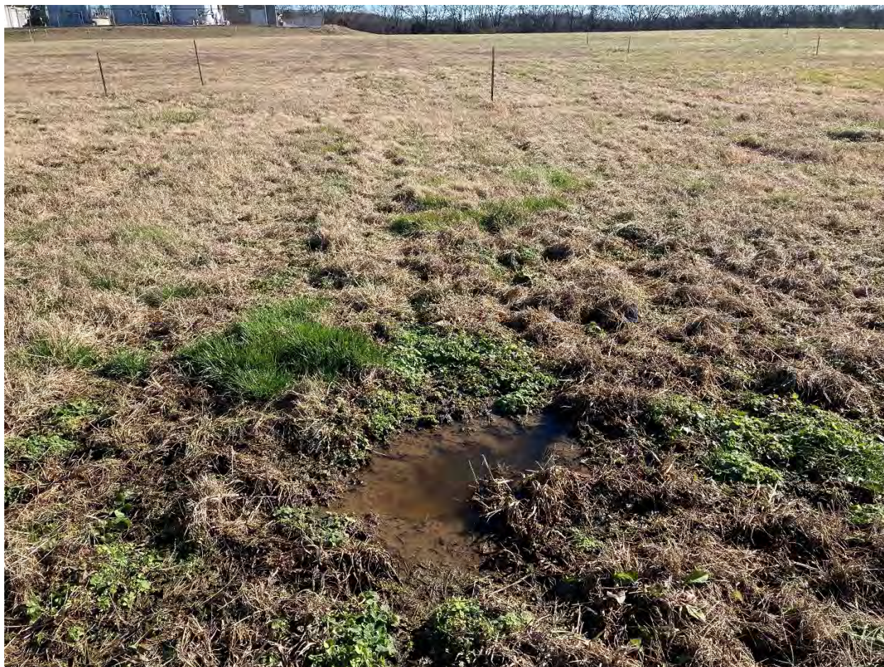
A2a. Localized saturation/ponding. Likely associated with a failed emitter or damaged line.
