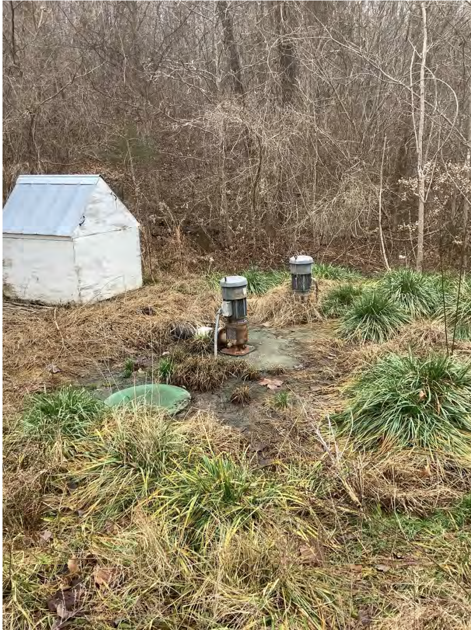
X2. Wastewater effluent being discharged from the pump vaults rather than to the drip field.
