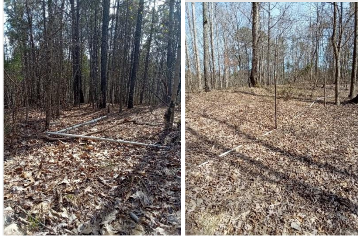
Exposed spray field distribution lines which have since been buried.
