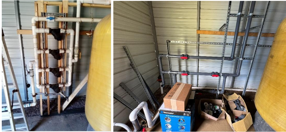
Strainer intended to capture larger solids before flow enters the sand filter before (left) and during replacement (right).
