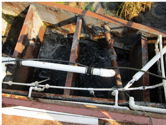
Leaking aeration lines, consisting of narrow PVC piping, throughout site.
