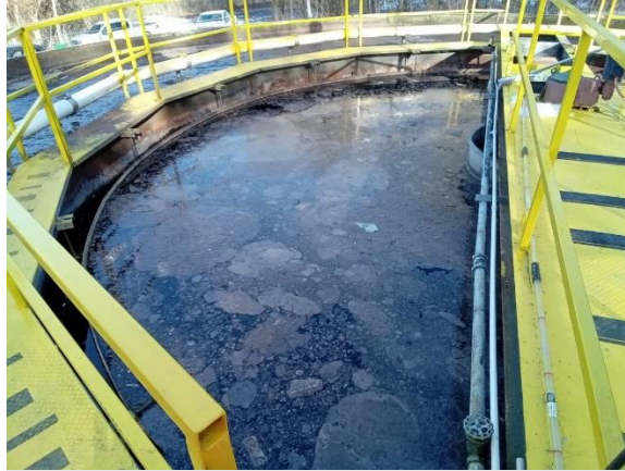
Example of new conduit installed across clarifier basin (narrow white piping above steel pipe).
