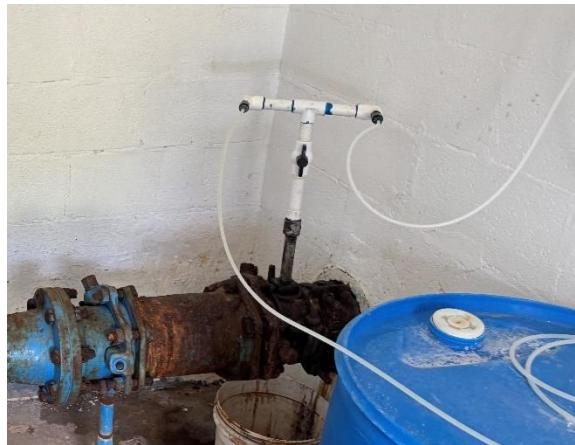
New chlorine injection port piping.
