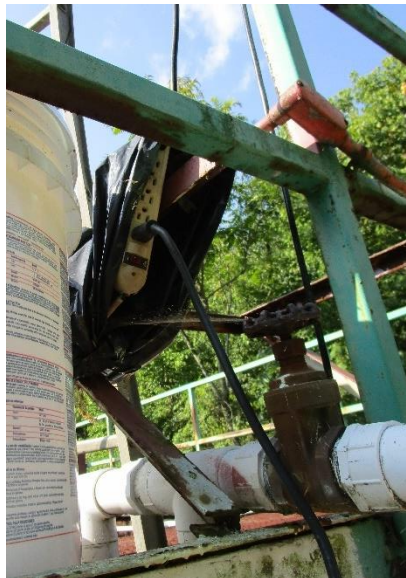
Improper power supply vulnerable to water infiltration from treatment processes and weather events.
