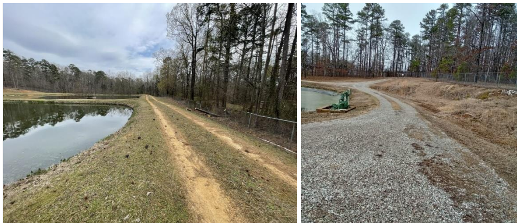
Typical lagoon driving paths before (left) and after gravel application (right).
