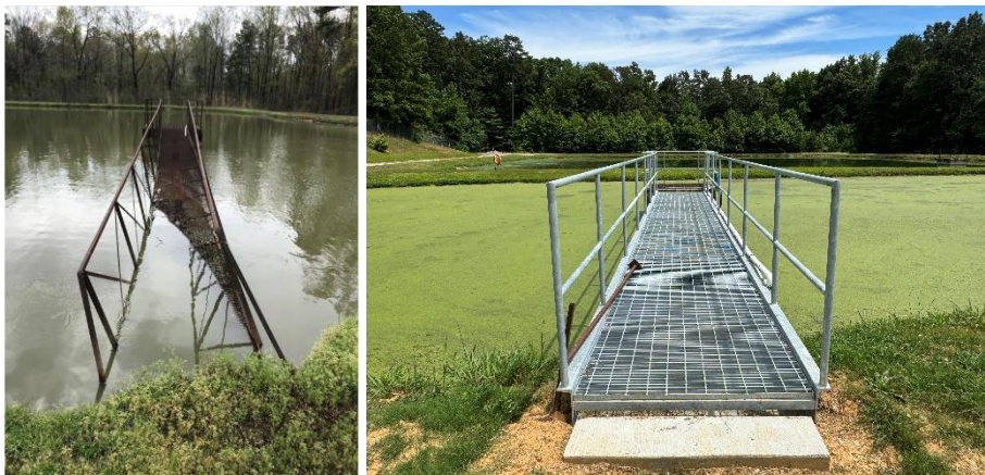
Failing catwalk structure before replacement (left) and after replacement (right).
