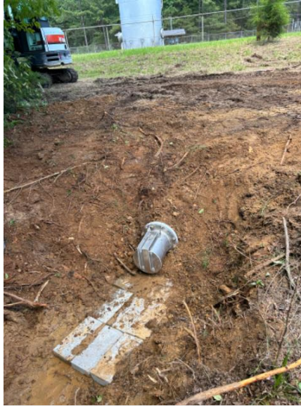
Vegetation cleared and new flap installed on drain line.
