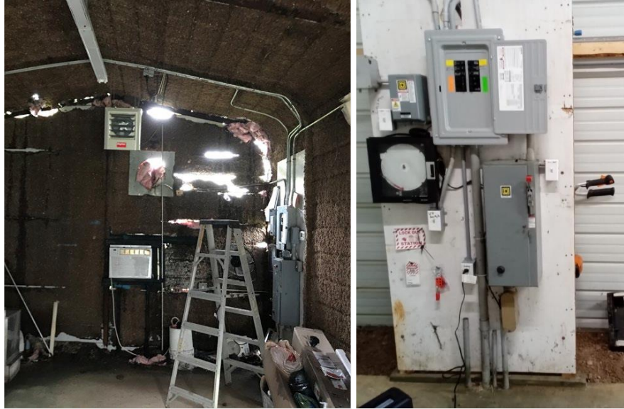
Poorly mounted power and control systems (left), remounted with rehabilitation of filter/disinfection shed (right).
