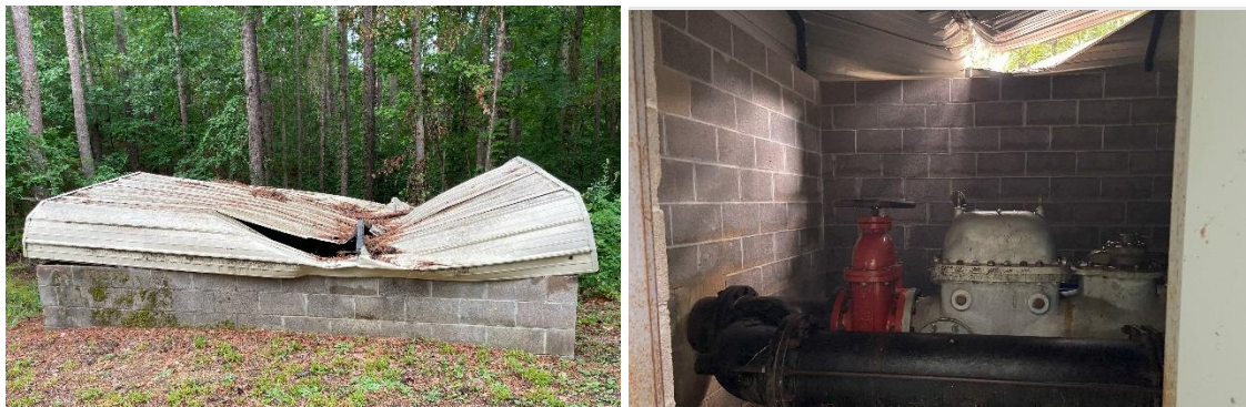
View of roof damage from the exterior (left) and interior (right).
