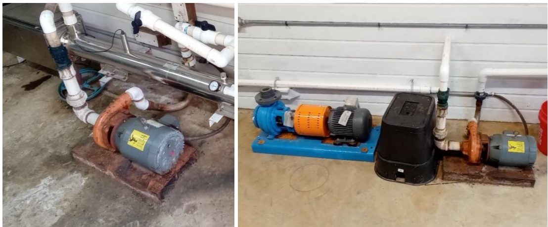
Single effluent pump present at acquisition (left), new backup effluent pump (in blue) now on site (right).
