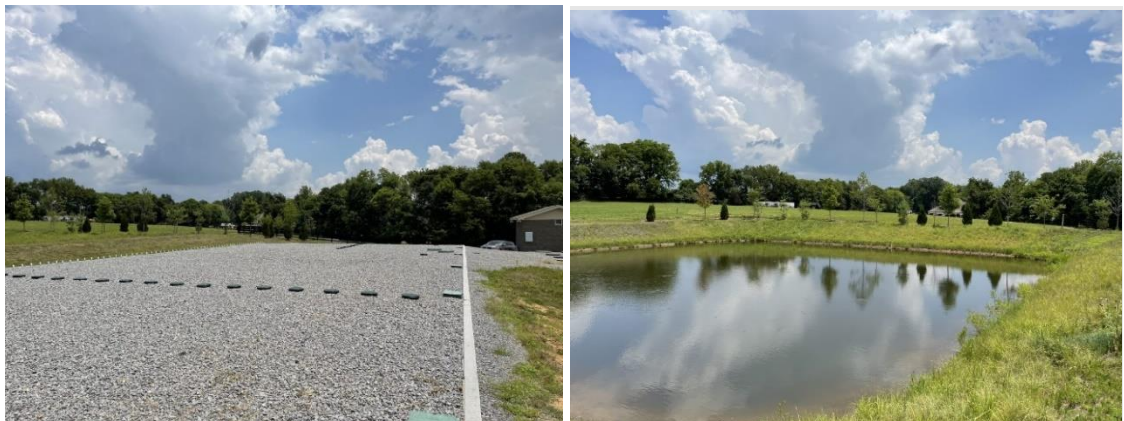
Sand filter and emergency storage pond.
