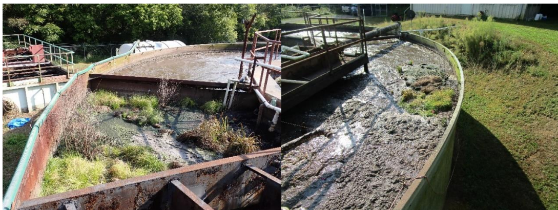
Rusting tanks, sludge accumulation, filter tanks(left).
