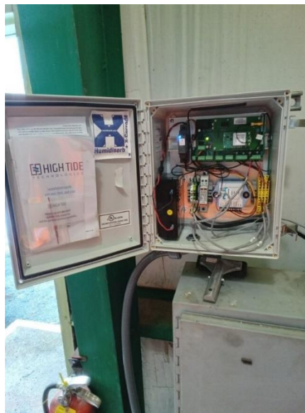
New remote monitoring unit at Grassland.
