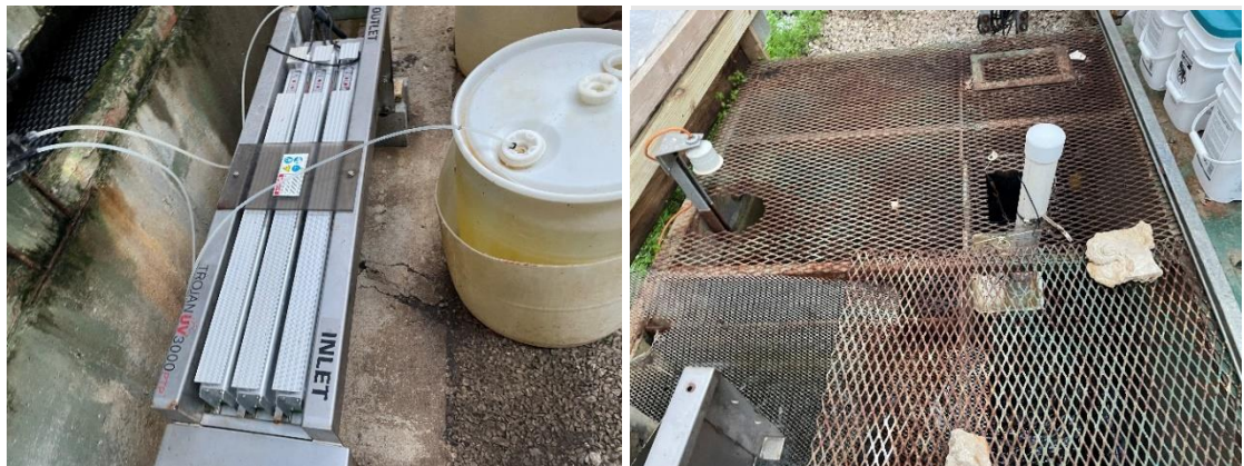
Ultraviolet disinfection (left) and secondary chlorination/dechlorination (right) disinfection systems.
