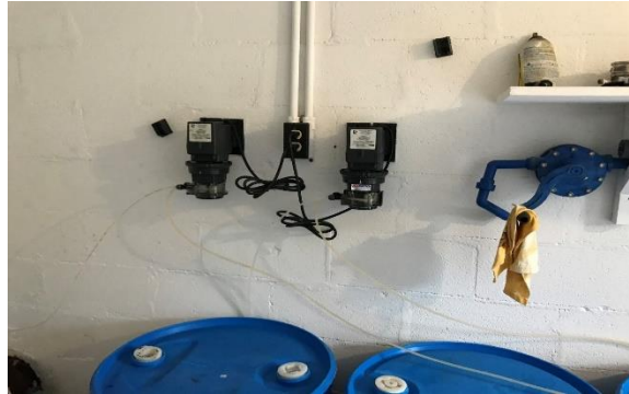
Chemical feed pumps and lines.
