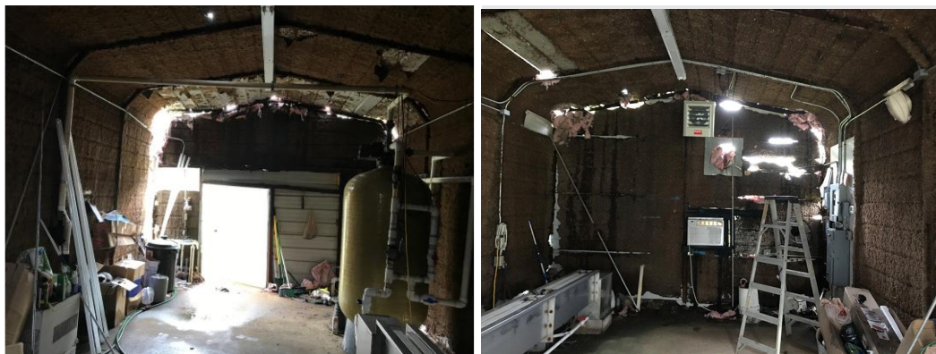
Severely deteriorated interior of filter and disinfection building.
