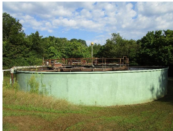
Grassland package plant tank – notice plants that had attached to debris.
