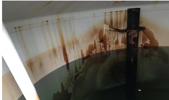
Sediment and rust staining on inside of tank prior to cleaning.
