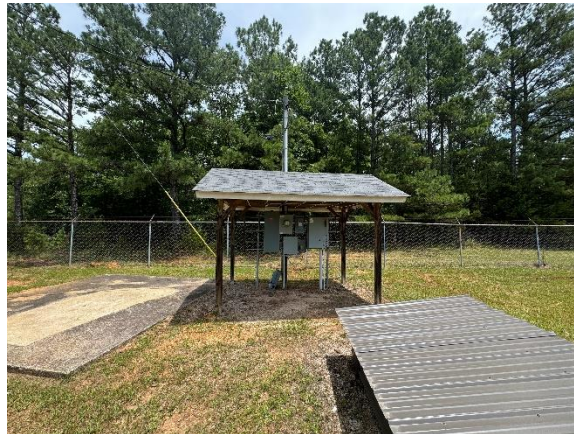
Concrete pad to the left of the power panels for future backup generator installation.
