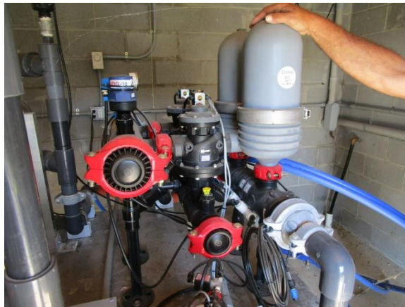
Pumping system for drain field.
