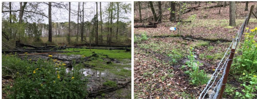
Overloaded spray field area due to inadequate size (left); runoff from spray field due to overloading (right).
