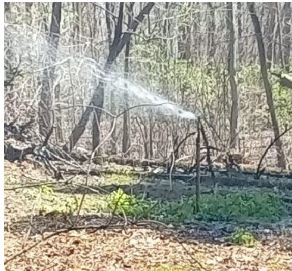
Example of spray field head.
