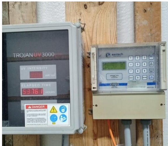
Recalibrated flow meter and UV intensity meter.
