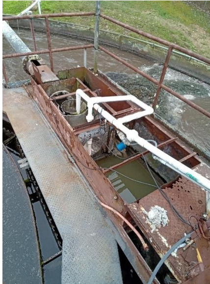
Loose wiring over treatment basins.
