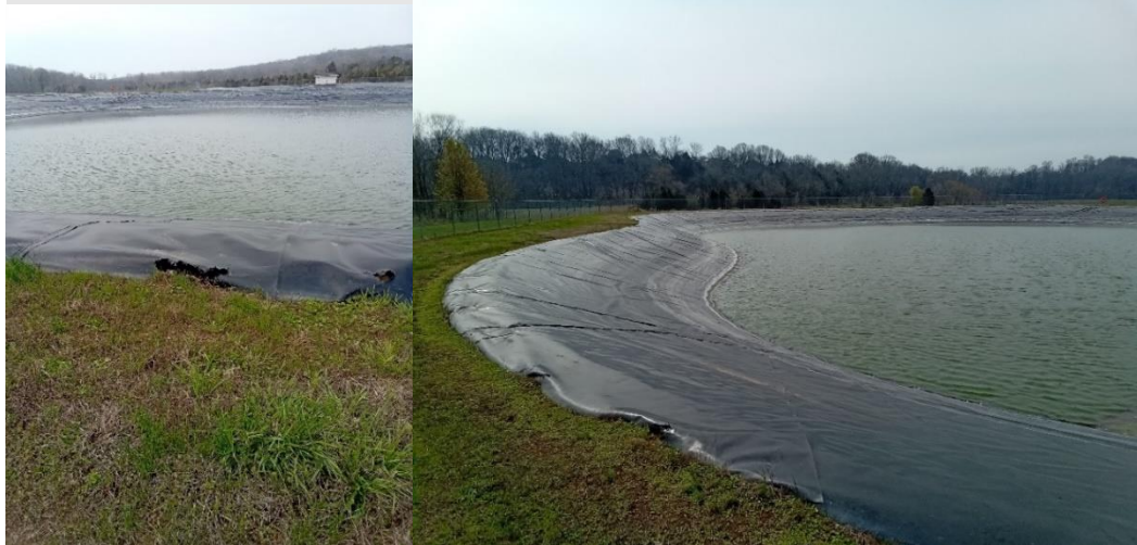
Section of lagoon liner damaged by animals (left) and repairs completed and liner re-tensioned (right).
