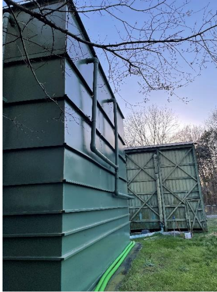
Anaerobic reactor (left) and nitrification tower (right).
