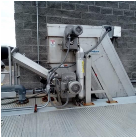
Screening system and compactor.
