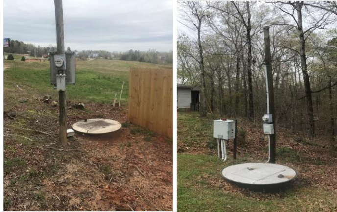
Typical lift station at Shiloh Falls.
