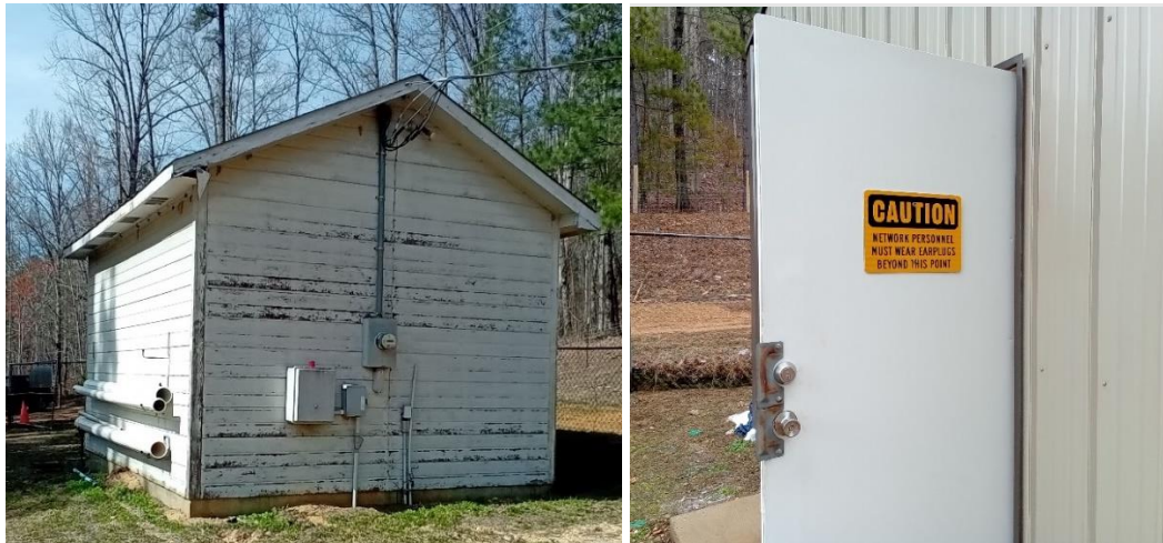
Blower building at acquisition with deteriorating roof and siding; new aluminum siding on blower building.
