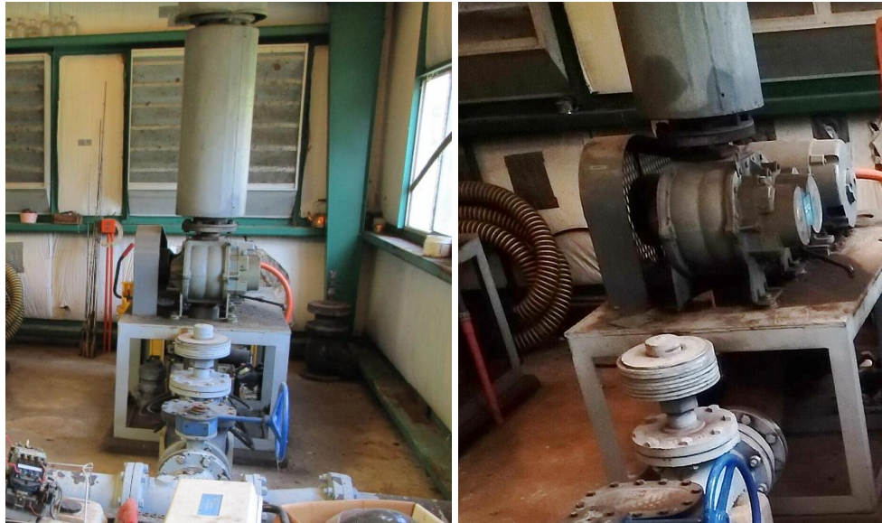
Failed blower at acquisition (left) and after motor replacement (right).
