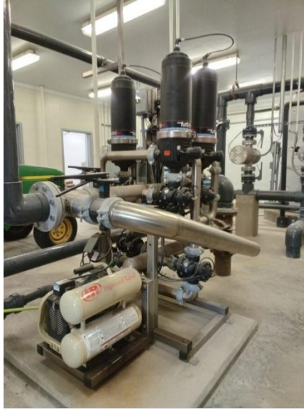
Turbo-disk filter system.
