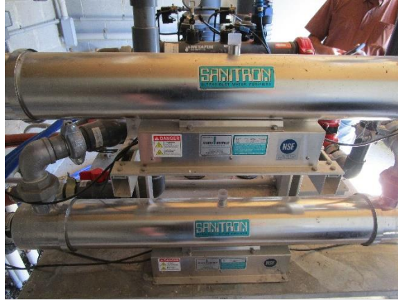
Ultraviolet disinfection system.
