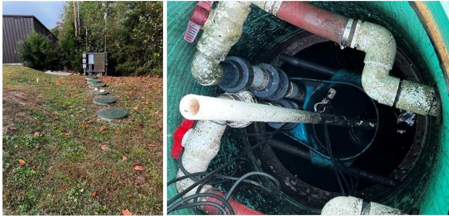
Septic tanks and part of the pumping system.
