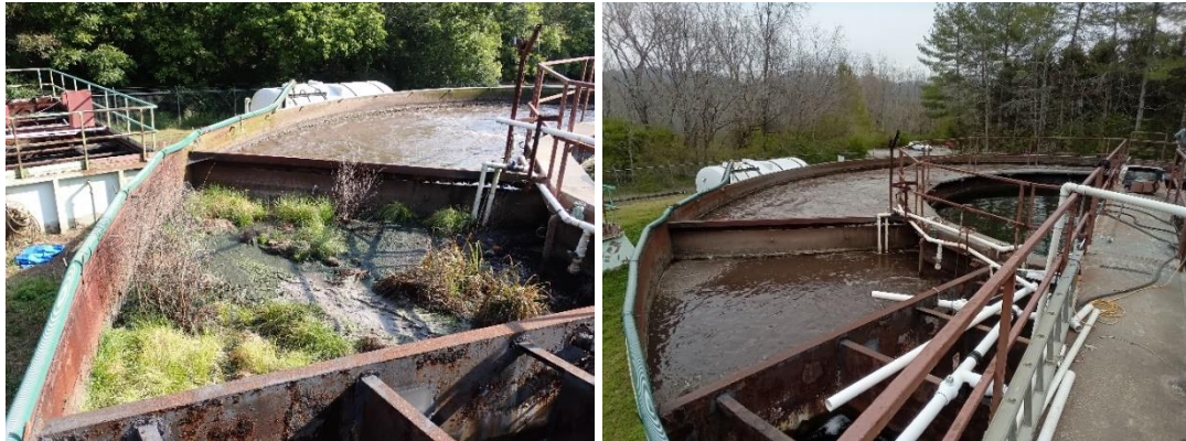
Floating sludge in aeration basins before (left) and after (right) clearing.
