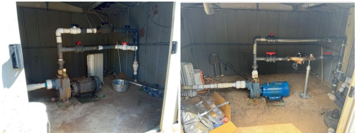
Discharge pump and motor before (left) and after (right) repair.
