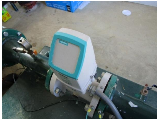
Repaired flow meter
