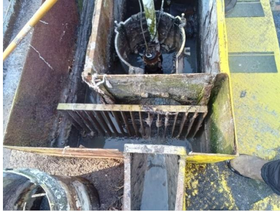
New bar screen for catching nuisance solids installed ahead of comminutor.
