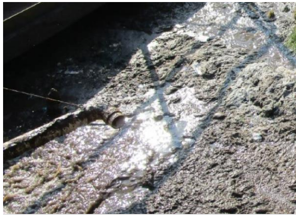
Blocked sludge return line.
