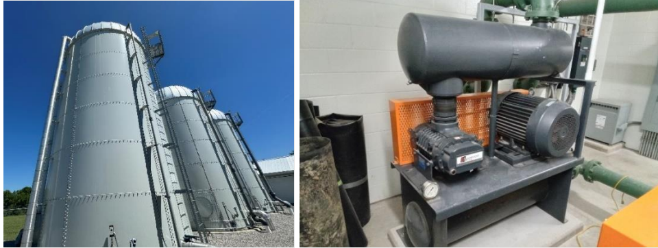
New aerobic and anaerobic Cambrian towers and part of the blower system with replaced VFD.
