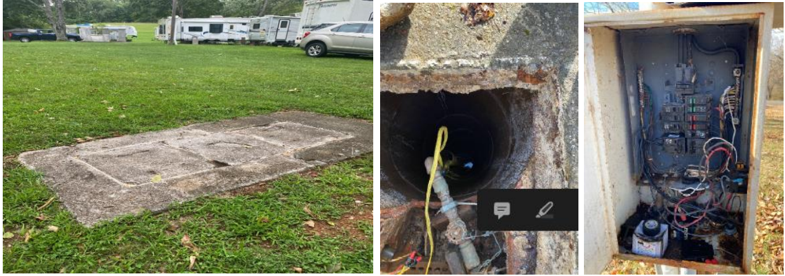
Well box (left), well interior (center), existing well control (right)
