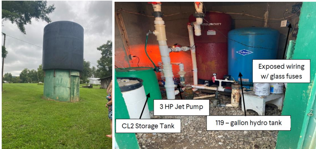
Existing storage tank and equipment located under the concrete stand.
