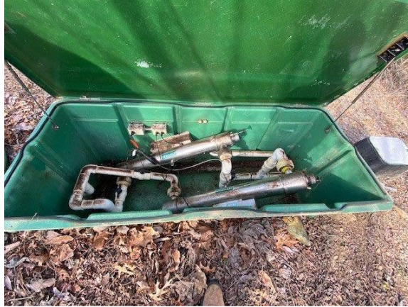
Out of service UV disinfection system
