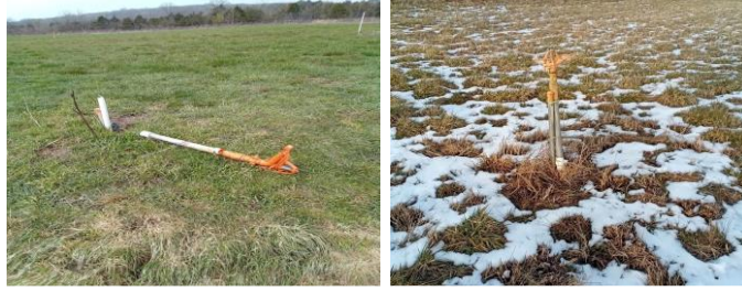
Broken (left) and repaired (right) spray field spigot.
