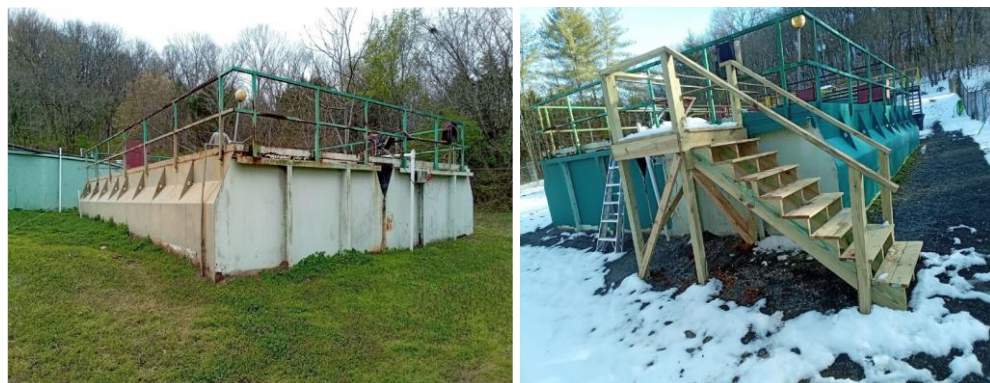
Package plant lacked permanent access, Operators used a temporary ladder (left), Permanent access installed (right).
