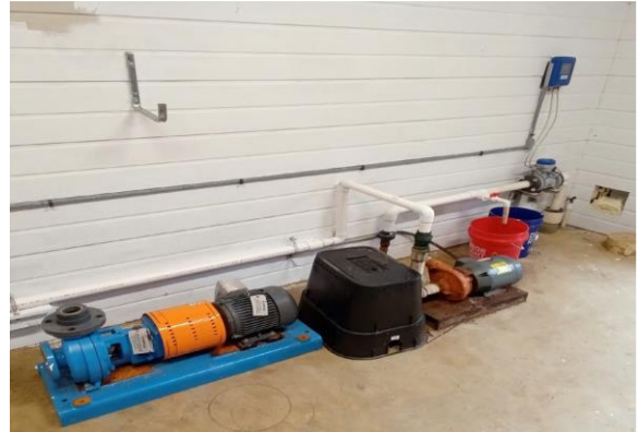
System lacking redundant booster pump to maintain minimum system pressure (left). redundant booster pump installed to maintain system pressure (right).
