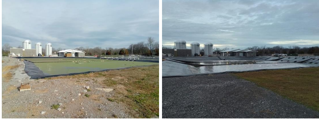
Prevalence of duckweed prevents proper treatment (left), duckweed removed, treatment restored.
