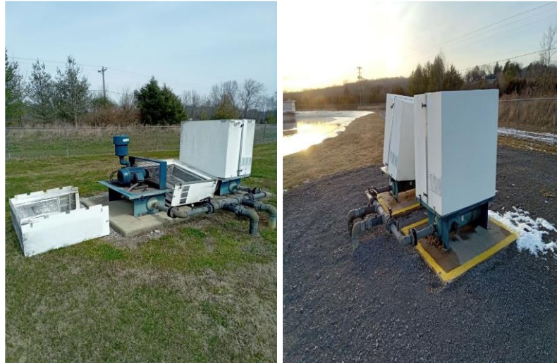
Unguarded blower, unsafe, grassy work surface (left). Blower box repaired, all weather terrain work surface installed.
