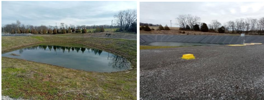
Hideaway lagoon lacked berm erosion measures (left), berm erosion measures installed.
