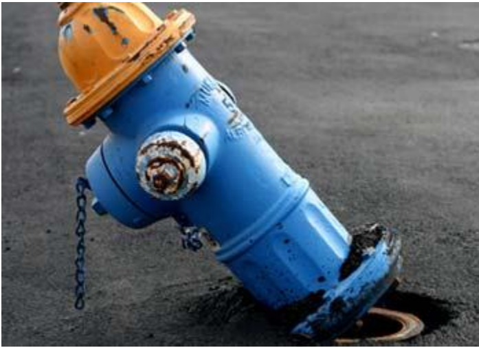
Dry-Barrel Hydrant
