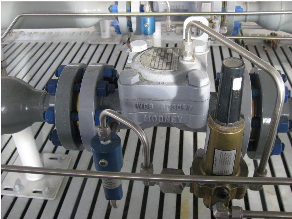
Account 379.00, Measuring and Regulating Station Equipment - City Gate Regulator
