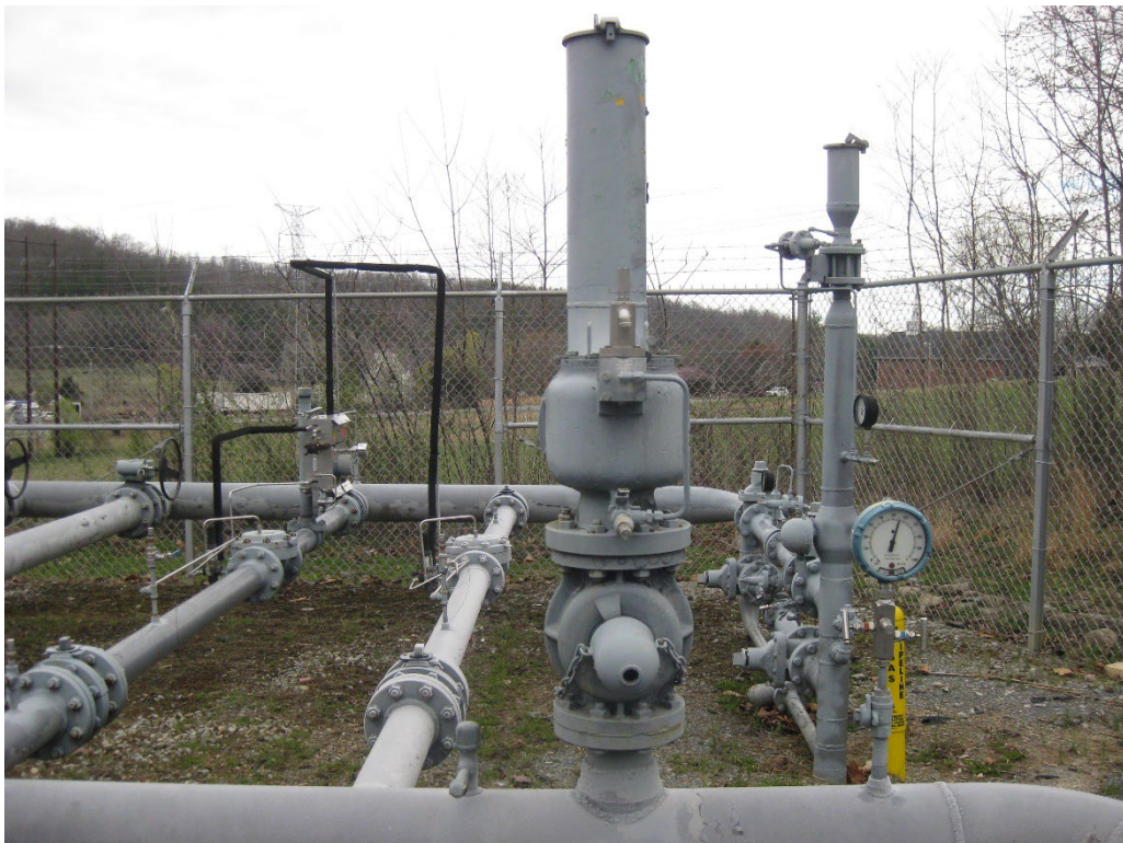
Account 378.00, Measuring and Regulating Station Equipment Regulator
