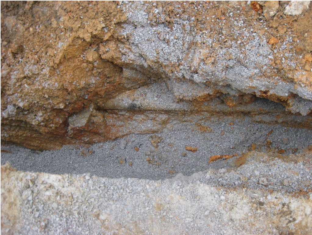
Account 376.00, Mains 2in Mains - Steel (Being Replaced)
