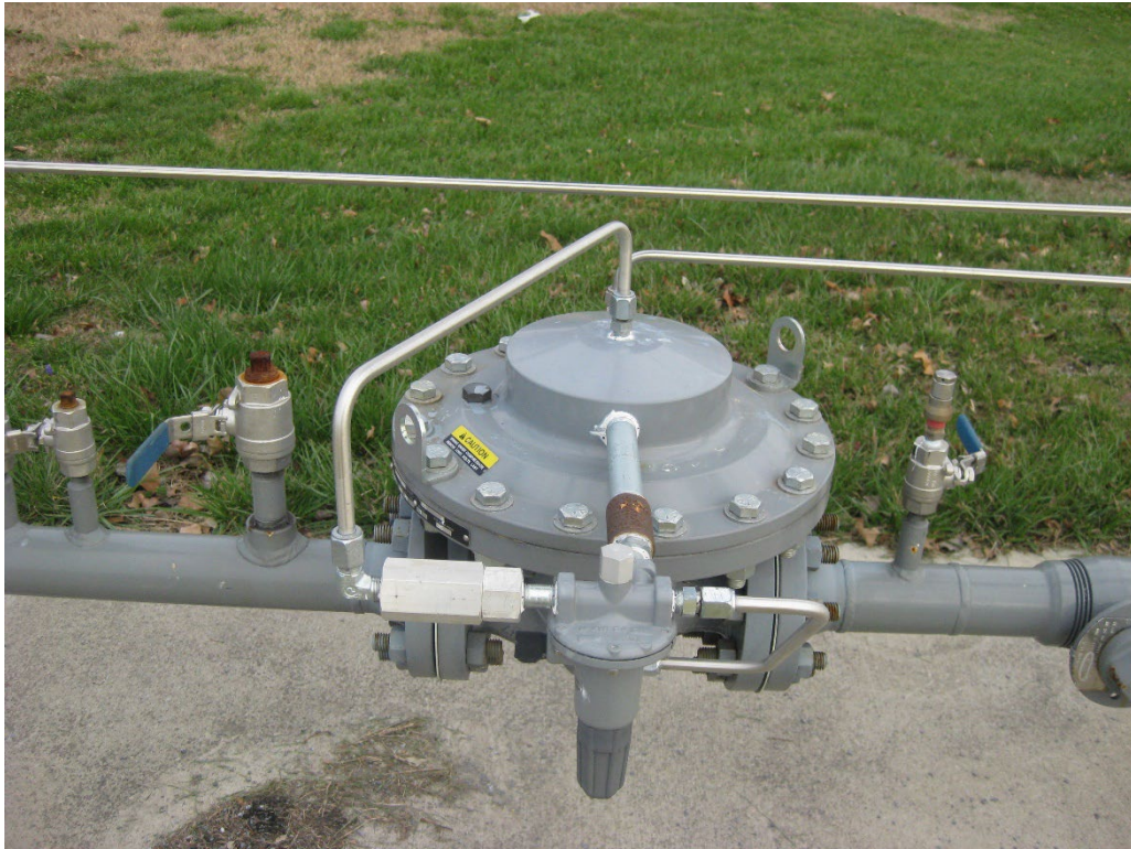
Account 378.00, Measuring and Regulating Station Equipment Regulator
