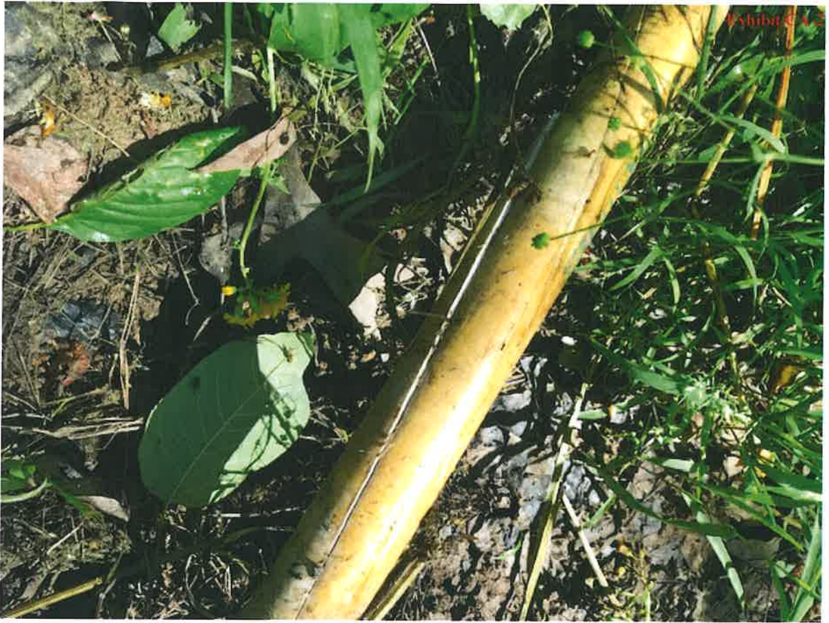
Image 11 - Broken spray field lateral. (Promptly repaired upon notification.)
