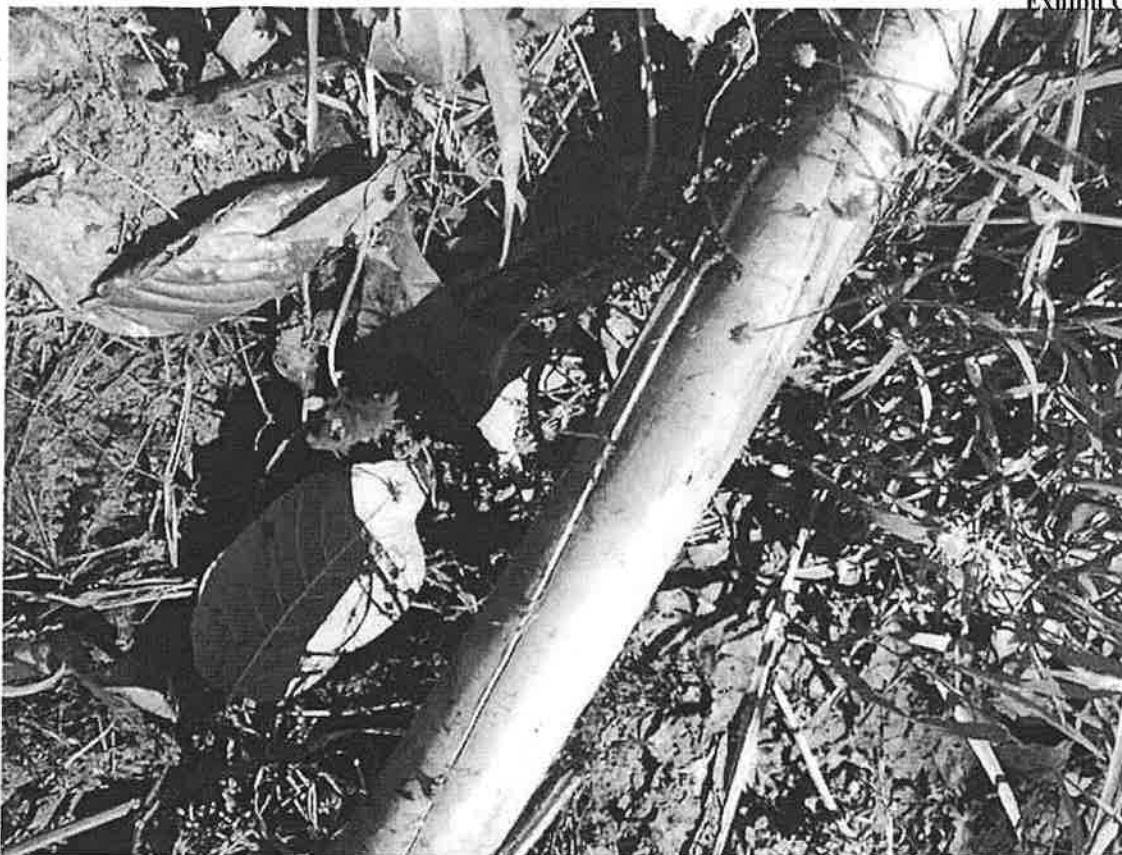
Image 11 - Broken spray field lateral. (Promptly repaired upon notification.)
