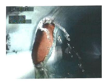
IDG recommends that any services on lines that are rehabilitated receive at least a "cut and buff / lateral seal" treatment
