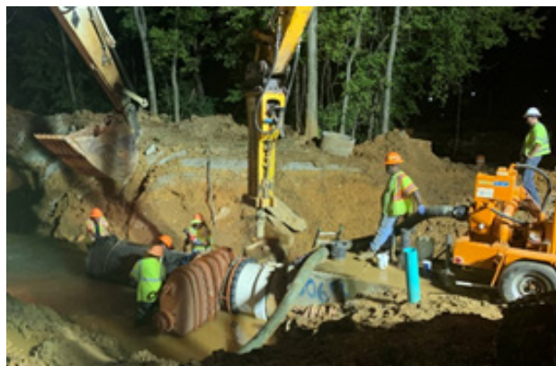
Crews Working on 36" Water Main Repair
