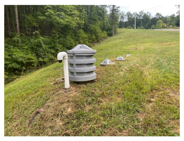
$8000\mbox{-}\mathrm{gallon}$  underground storage tank fed from the lower pump station and into the upper pump station.
