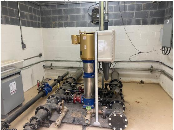
Interior of upper pump station. Two 480V 3 Phase 30 hp pump motors with room for future expansion to a third pump if needed.
