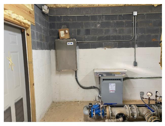
Lower pump station 115V step down transformer and circuit panel.
