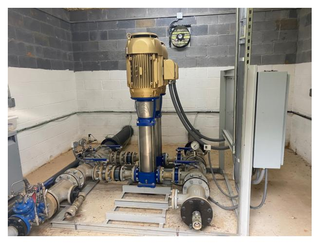
Interior view lower pump station. Two 480V 3 Phase 50 hp pump motors with room for future expansion to a third pump if needed.
