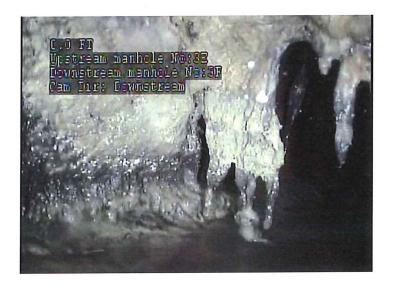
3. Manholes can be a major source of I/I, and in some cases may need to be replaced entirely. One or two manholes near Sonic in the Grassland Commercial Area are in need of repair or possible replacement, along with manholes in front of Grassland Middle School. Grouting and sealing with cementitious or epoxy coatings might work, but if the manholes are structurally deficient, replacing them altogether could be necessary.
