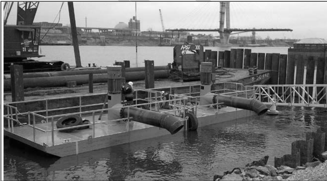
Figure 2 Alternative 1, Phase 1 – Floating Pump Station
