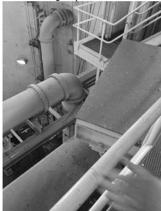
Discharge Pipe Wall Penetration
