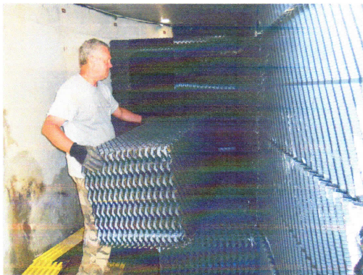
ABOVE: Dart Kendall stacks the media blocks (Brentwood Industries) four high in the treatment tank, leaving 12 inches of clearance at the top. RIGHT: Cliff Kendall buries drip tubing 9 inches deep using a Caterpillar 226 skid-steer loader with Bradco trencher (Paladin Construction Group).
