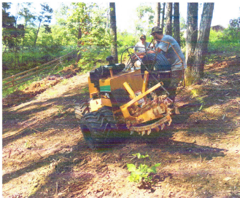
Cliff Kendall (right) and Barry Little install Geoflow drip tubing using a modified LM42 Vermeer walk-beside vibratory plow with 50 hp turbo diesel. The plow has dual wheels on the downhill side.
