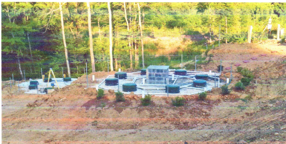
At the left, the 35,000-gallon poured-in-place circular dosing tank; at the right, the treatment tank with shrubs planted around it. (Photos courtesy of Dart Kendall)
