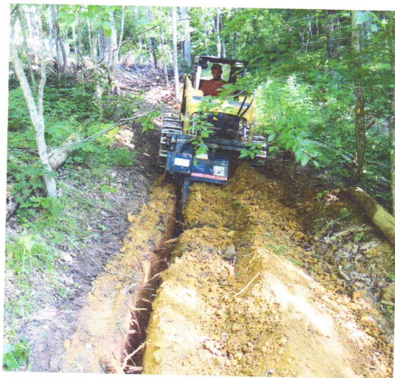
ABOVE: Dart Kendall stacks the media blocks (Brentwood Industries) four high in the treatment tank, leaving 12 inches of clearance at the top. RIGHT: Cliff Kendall buries drip tubing 9 inches deep using a Caterpillar 226 skid-steer loader with Bradco trencher (Paladin Construction Group).
