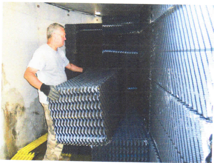
ABOVE: Dart Kendall stacks the media blocks (Brentwood Industries) four high in the treatment tank, leaving 12 inches of clearance at the top. RIGHT: Cliff Kendall buries drip tubing 9 inches deep using a Caterpillar 226 skid-steer loader with Bradco trencher (Paladin Construction Group).
