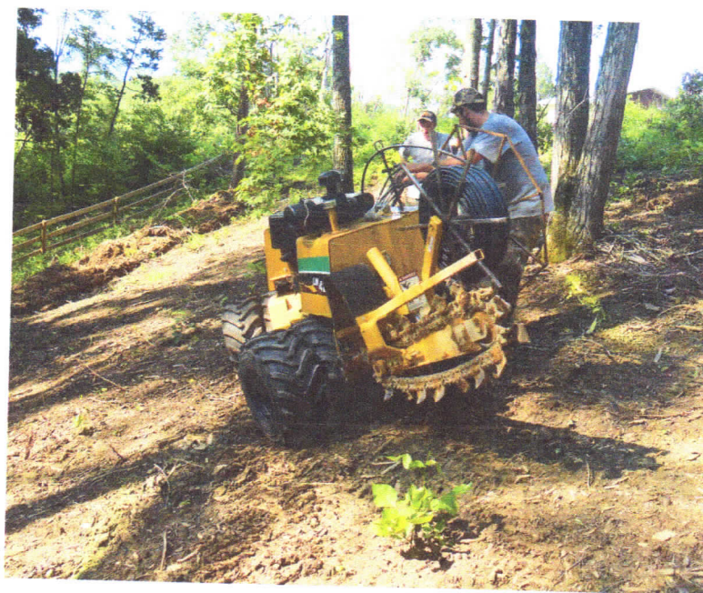
Cliff Kendall (right) and Barry Little install Geoflow drip tubing using a modified LM42 Vermeer walk-beside vibratory plow with 50 hp turbo diesel. The plow has dual wheels on the downhill side.
