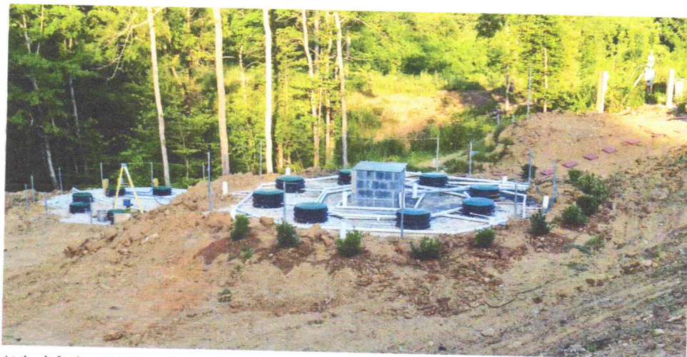
At the left, the 35,000-gallon poured-in-place circular dosing tank; at the right, the treatment tank with shrubs planted around it. (Photos courtesy of Dart Kendall)
