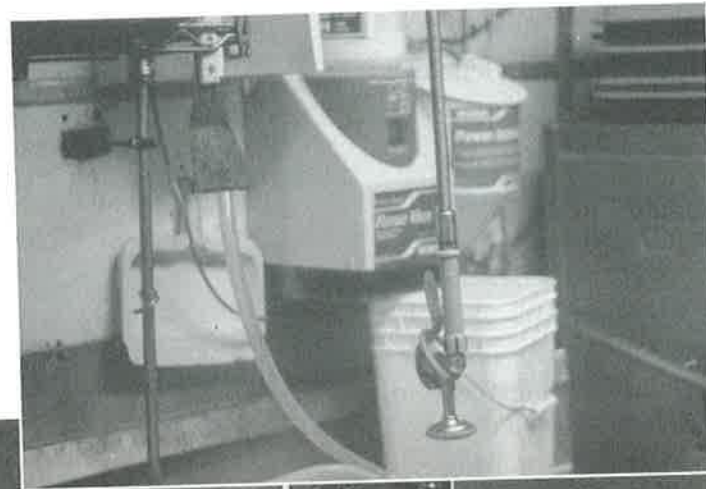
Figure 4.12 Dishwashing operations that use an automatic shutoff sprayer for pre-rinsing can save water compared with methods that rely on constantly flowing faucets and rinse tanks. (Photo courtesy of Amy Vickers & Associates, Inc.)
