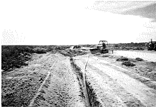
Figure 4: spoolable pipe being pulled down right-of-way by bulldozer
