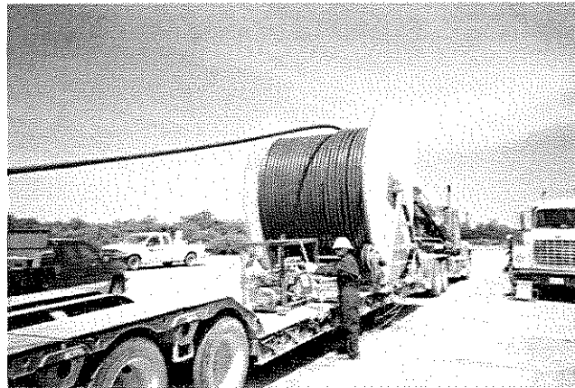
Figure 3: 3-in., 1,500 psig spoolable pipe
