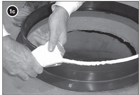
MA320 adhesive on bolt-down riser lid adapter
