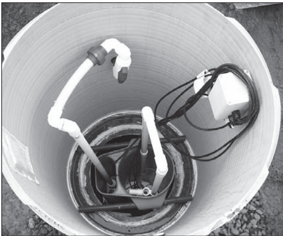
When the union is disconnected, there should be enough clearance to allow removal of the vault.
