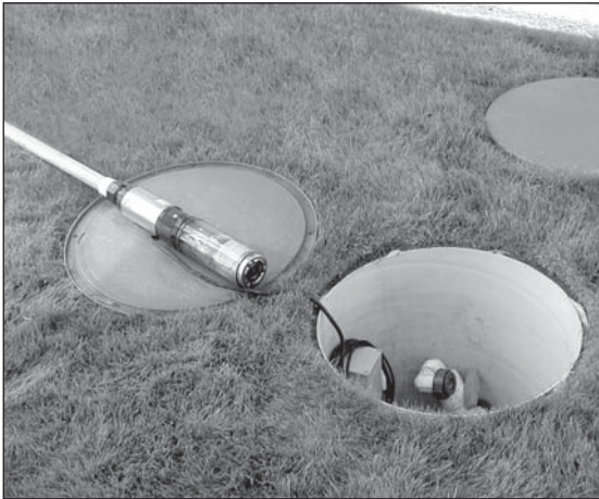
The pump can be removed without disconnecting the power cable.
