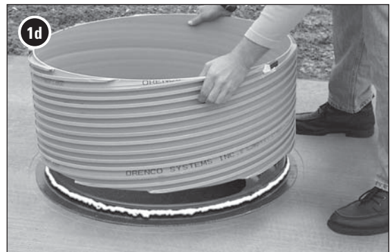
MA320 adhesive on bolt-down riser lid adapter
