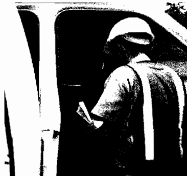
Above: Crew inserts CCTV camera for routine inspection of residential sewer line
