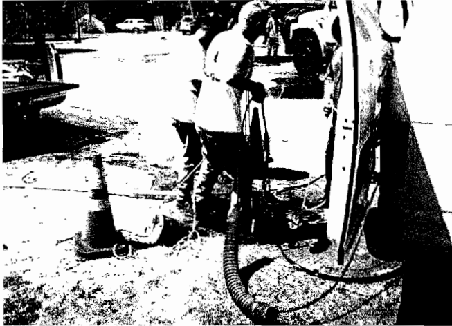
Above: Crew inserts CCTV camera for routine inspection of residential sewer line
